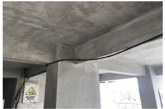
Gambar 13. Hasil Pengecoran Bekisting Aluminium
