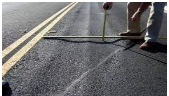
Gambar 3. Alur ( Rutting ) [13]
