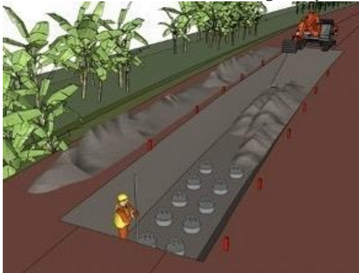
Gambar 2. Galian kepala tiang bore pile
