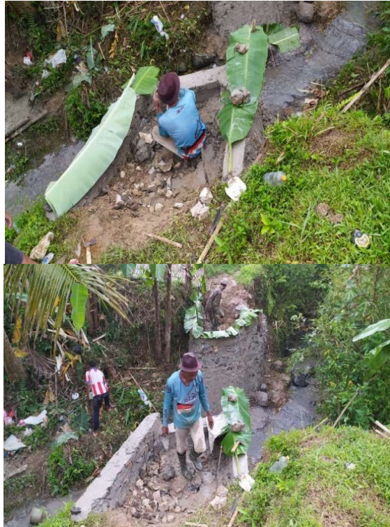
Gambar 9. Proses perawatan abutment
