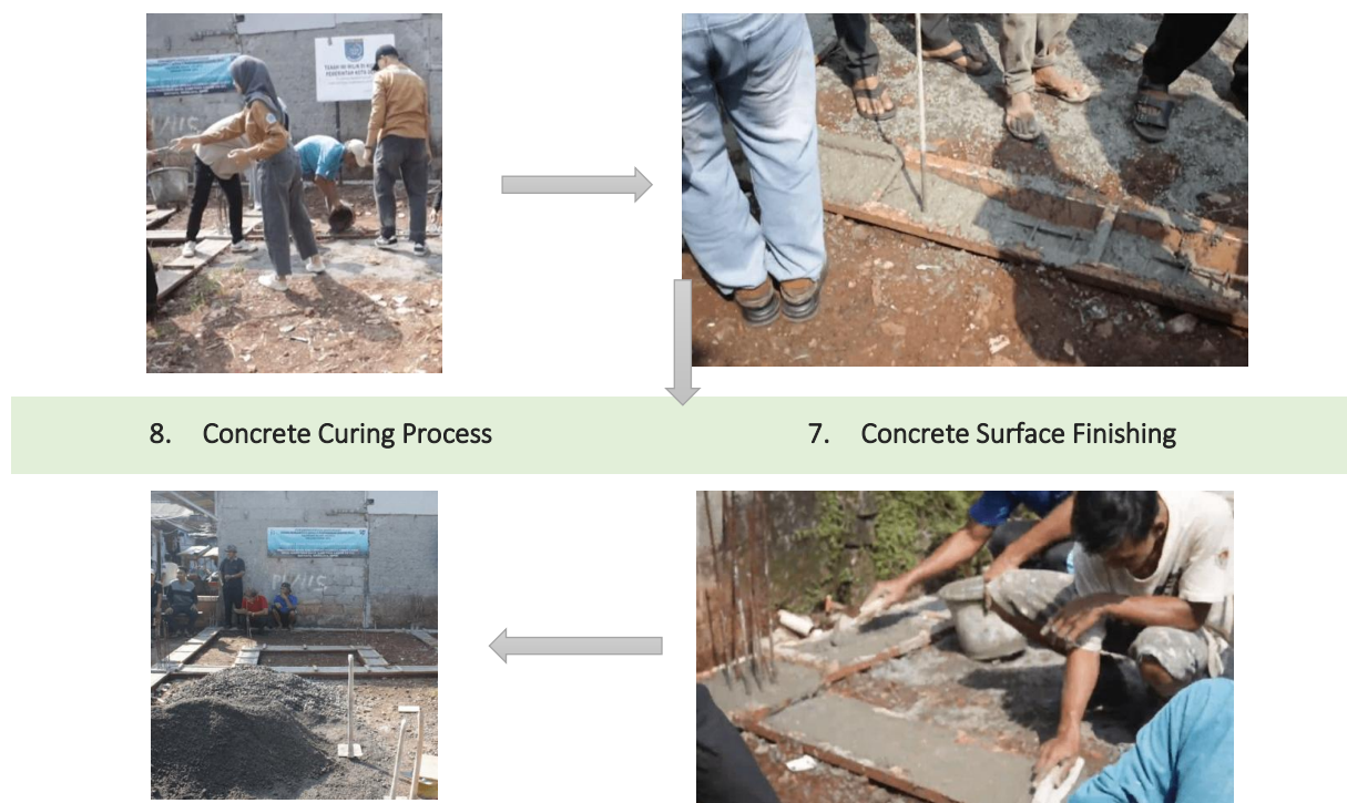
Figure 4. Stages of community service work in making SCC concrete blocks
