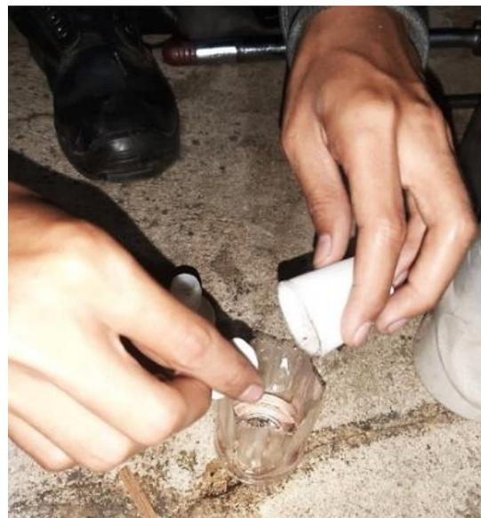
Figure 7. The process of mixing resin and catalyst
