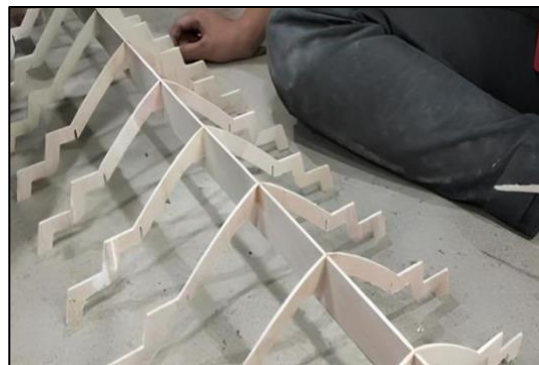
Figure 5. Assembly of the hull frame
