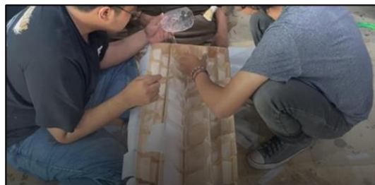
Figure 7. Clear resin coating
