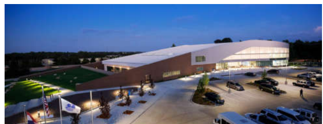
Gambar 7. Atap Maryland Heights Community Recreation Center
