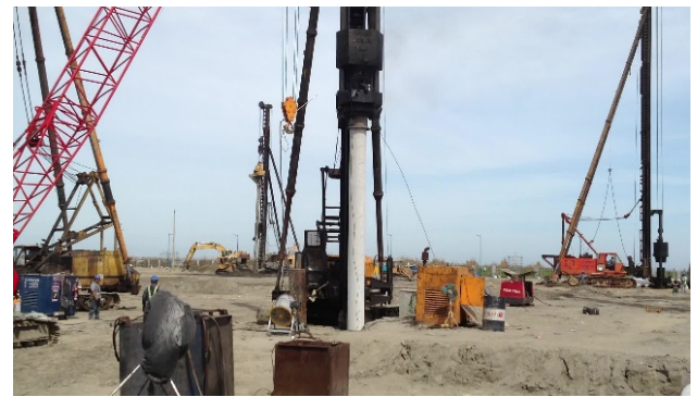
Gambar 1. Alat Pancang Diesel Hammer
