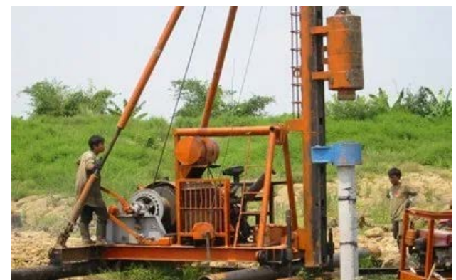
Gambar 2. Pile Driver Drop Hammer
