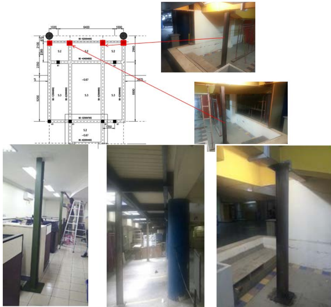
Figure 4. Temporary strengthening of the basement floor
