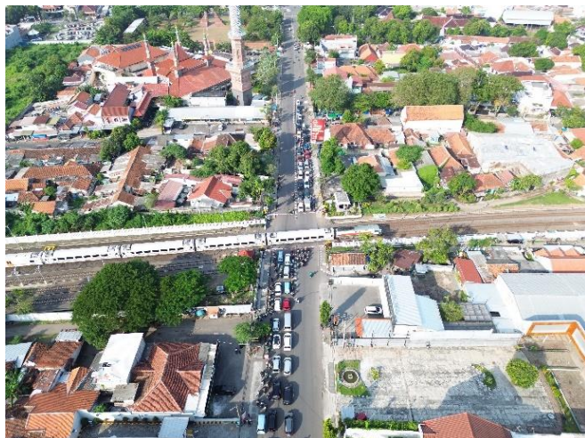
Figure 1. Traffic Phenomena at Level Crossing
